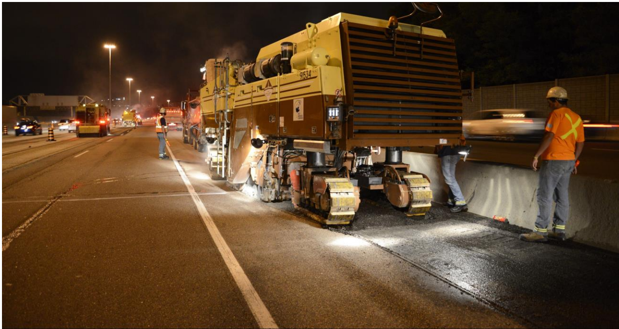
Nighttime paving on highway. Image courtesy The Miller Group.
