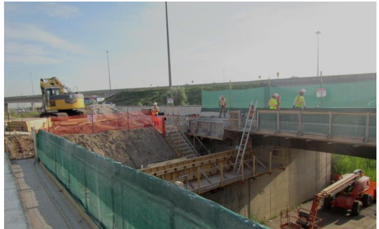
Excavation at the Steeles Avenue Overpass to Prepare Bridge Expansion
