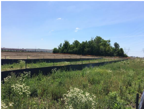
Wired Back Silt Fencing for Sediment Control
