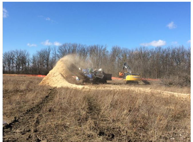
February 26, 2018. Clearing operation north of Langstaff Rd. Grinding of tree material. Some of the wood chips will be spread on the ground to reduce erosion.
